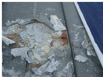
Result of using a hybrid roof.
